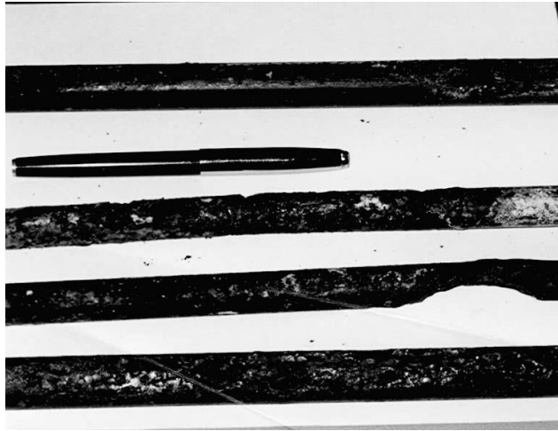
Figure 1.3 Reinforcing bars taken from under the end of a waterproofing membrane. They have been subjected to low oxygen conditions and therefore one of them shows severe local wasting. There was no expansive oxide growth.
